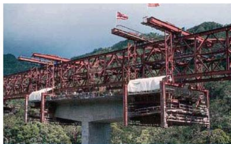
H-3 North Halawa Valley Viaduct - Hawaii (1990-1992)
