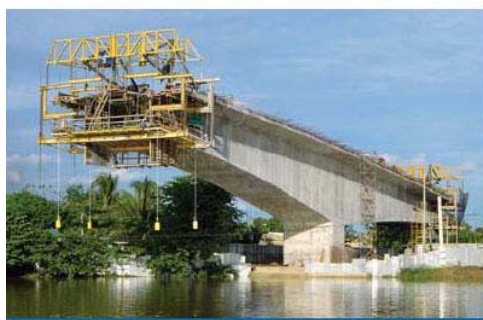
Sinu Bridge - Columbia (2005) 150m of main span length, 2 cantilevers
