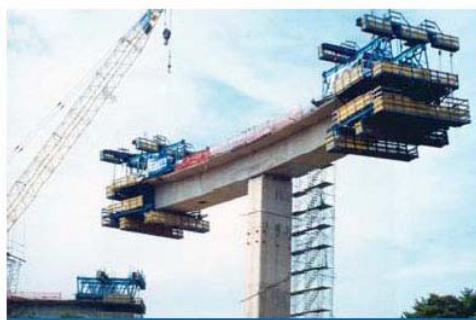
Ma Wan - Hong Kong (1999) 48m of main span length, 15 cantilevers
