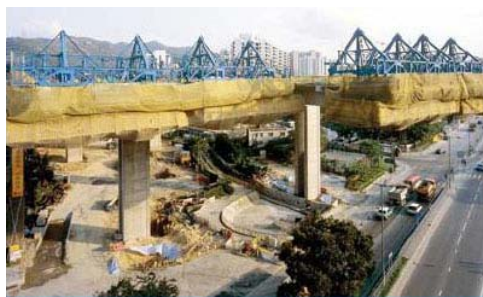
Deep Bay Link - Hong Kong (2004-2005) 71.5m of span length, 28 cantilevers
