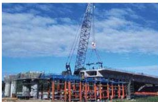
West Link - Australia (2004-2005) 86,000m 2 of deck, 3,013 segments
