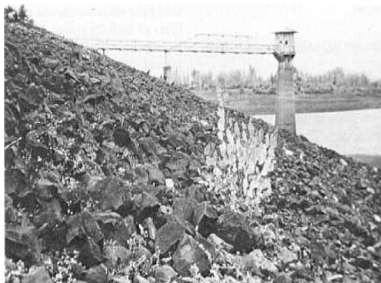
Figure 6-46.—Riprap on upstream slope of an earthfill dam. Dam is in excellent condition after 50 years of service. The structure is Cold Springs Dam, which forms an offstream reservoir on the Umatilla Project in Oregon. IO-2194.
